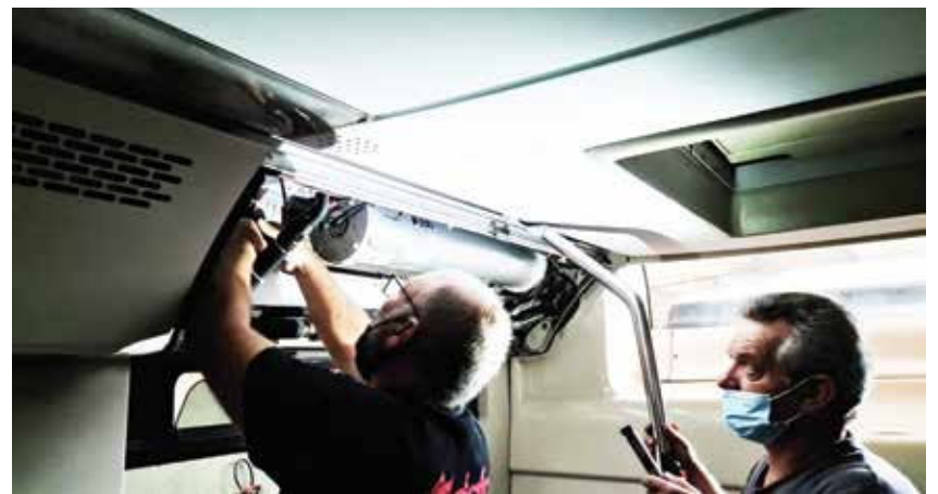
Installing Dafo's fire extinguisher
